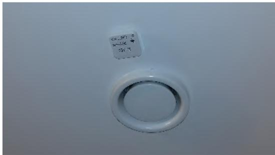
(a) Wireless Sensor Tag at Bathroom
